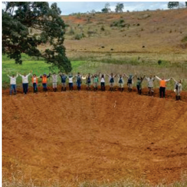
Figure 5: Implementation of barraginha. Retains rainwater and facilitates water infiltration into the soil, helps prevent siltation and control erosion. Source: https://refloresta.institutoterra.org/terradoce .
